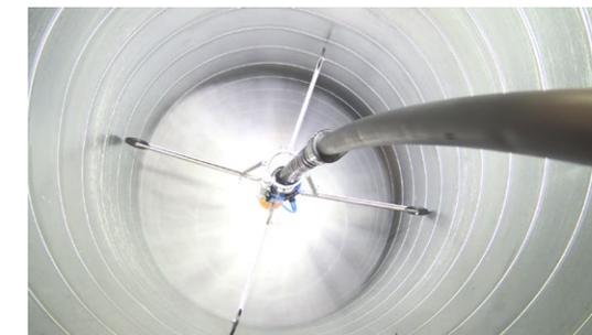
The centering device fixes the brush in the center of the duct.
